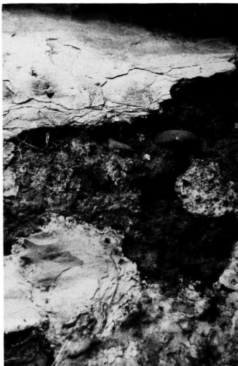
Fig. 22 (left) Coats of limewash applied to a pre-smoothed clay wall-face
