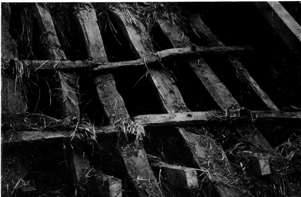
Fig. 52 Rafters at Lamonby Farm Cottage in long view and close-up, 1981
