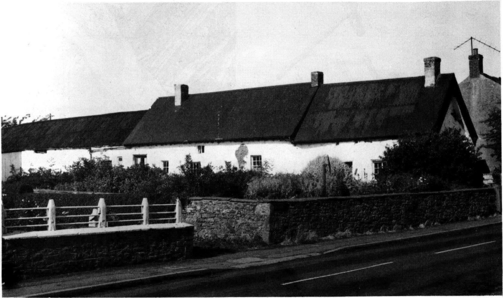
Fig. 56 Lamony Farm, fully roofed in galvanized iron, prior to rehabilitation in 1979
